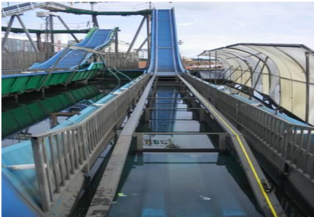
Splash tank and rails
