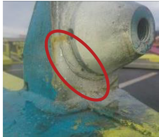
▲ Reverchon Crazy Mouse support column track allocation cone cracking
