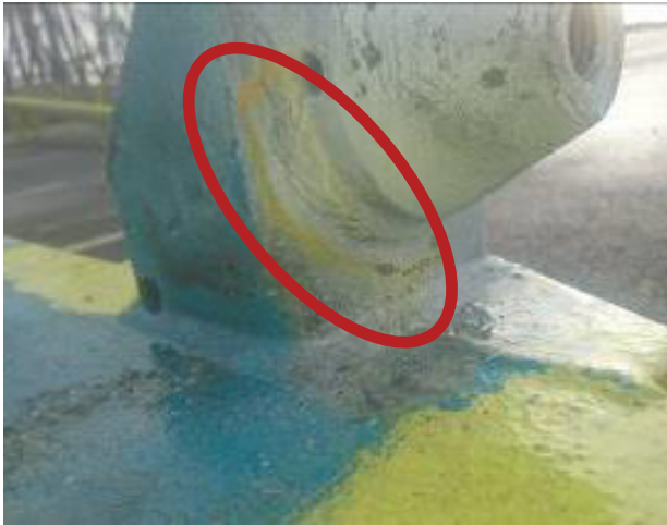
▲ Reverchon Crazy Mouse support column track allocation cone cracking
