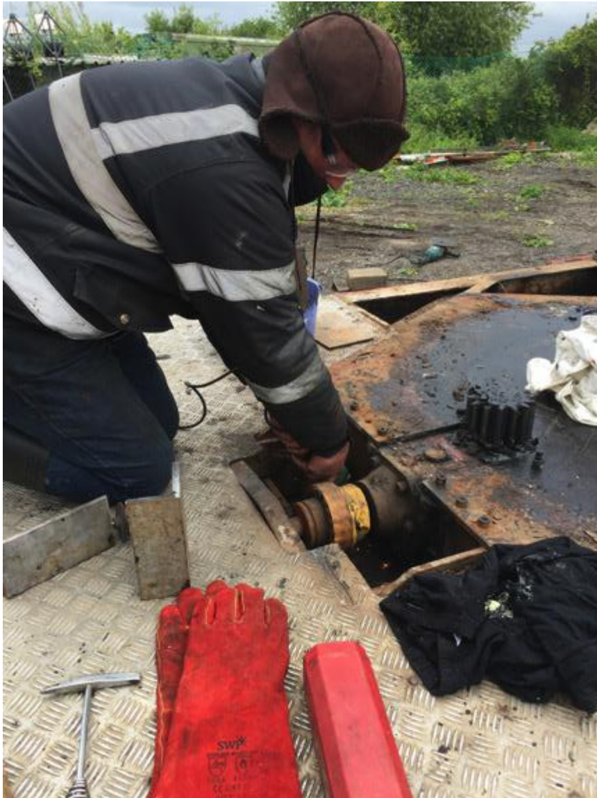
Above can be seen the six Allan key studs securing the gearbox and drive pinion. They had all sheared and could be lifted out by hand.
