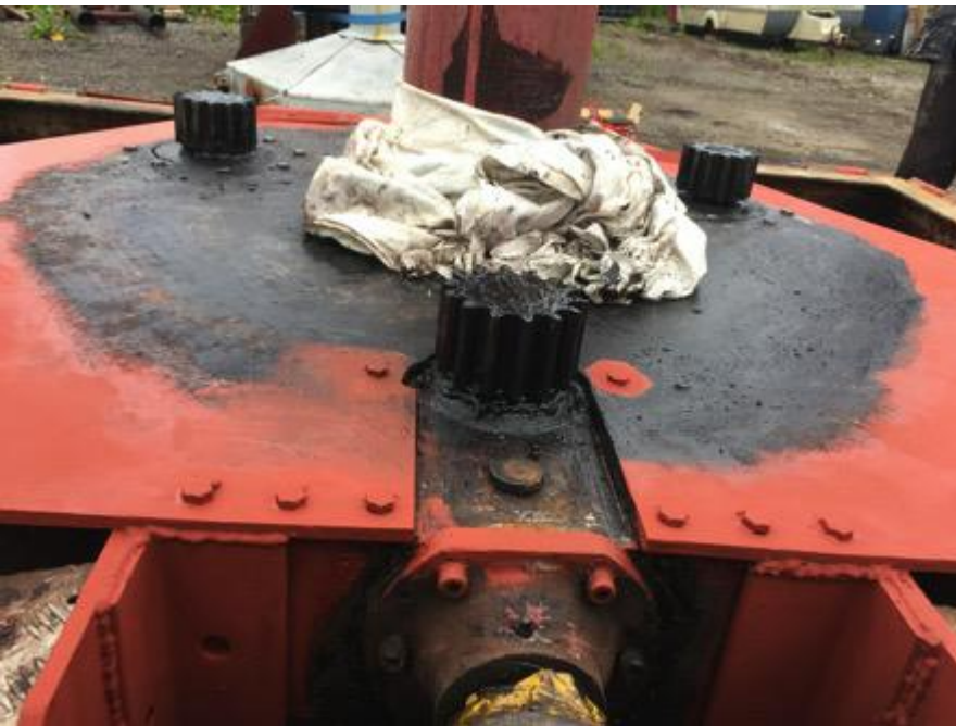
Two additional steel plates (angle steel) have been welded into the chassis to give additional support to the gearbox against the twisting movements created during ride acceleration.
